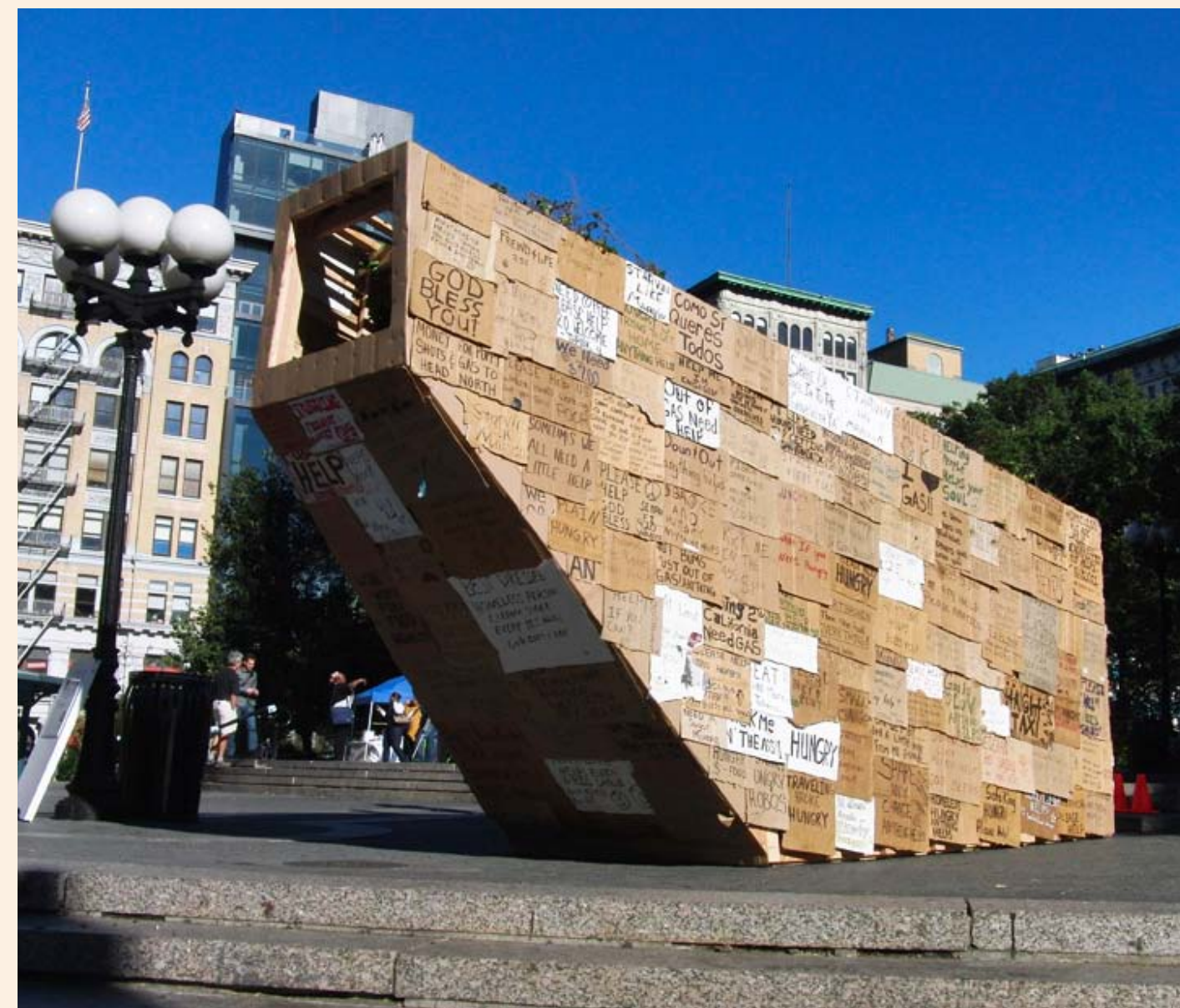
The final result was shorter than the initial 5.5-m-tall design, as the New York City Building Code restricted the height to 3 m. To maintain the original intent of framing the sky, the architects turned the structure on its side.
